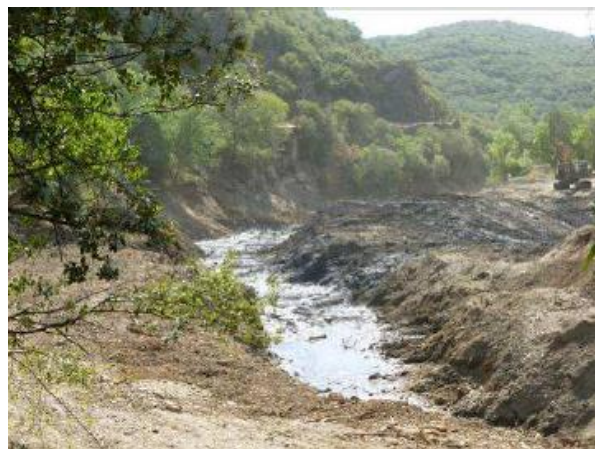
Removal of Biconque dam (6m high) in Lamalou on Bitoulet river in 2017, following the 2014 flood and safety concerns
