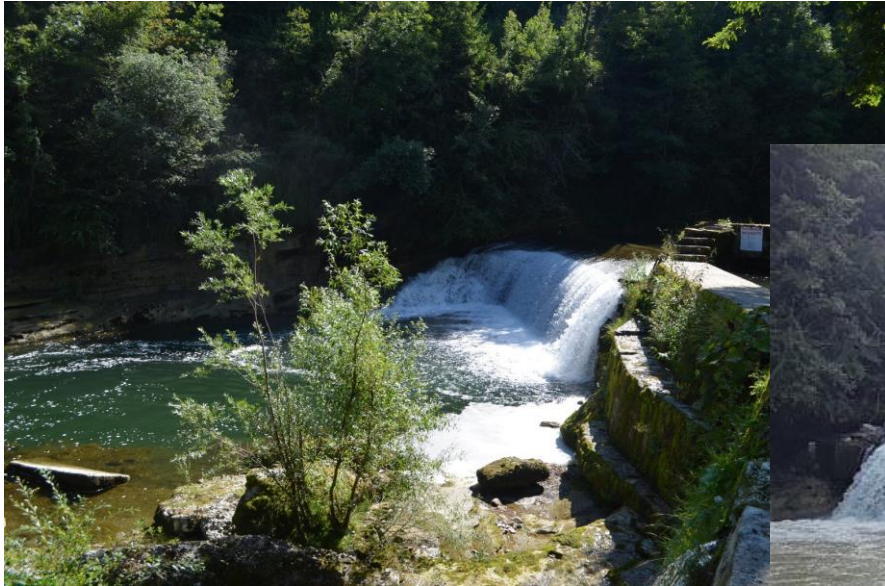
Removal on the Chéran river : Aumône weir in 2020 (4m high)
